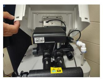
4. Install the bypass assembly using the two large black clips.
