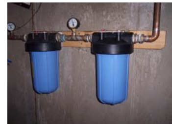
Two-stage big blue filter for home. First stage is 50 micron, second stage is dual-grade 25/1 micron filter.
