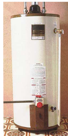
Water heaters can accumulate sand rust and sludge. If the water heater is corroding 'sediment' can actually be introduced into the water.
